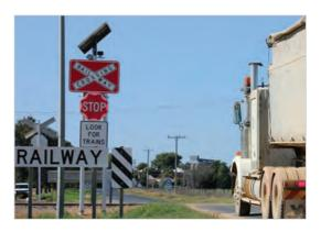
The trial radar-activated LED signs are designed to boost level crossing visibility for motorists:
